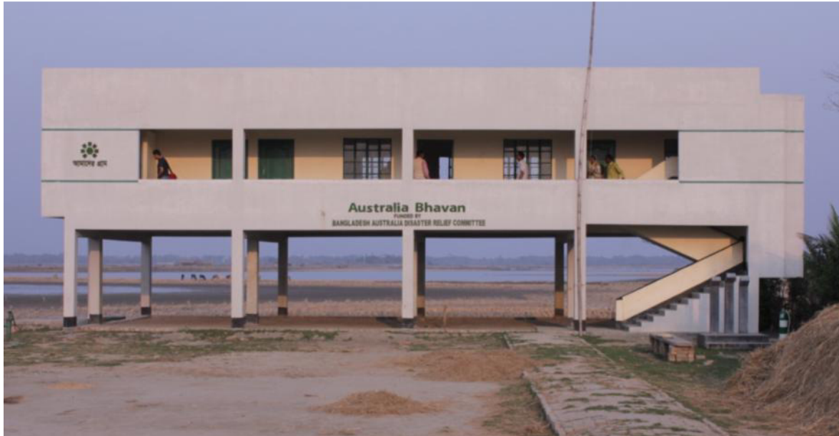
Completed School-cum-Cyclone Shelter named as AUSTRALIA BHABAN funded by BADRC
